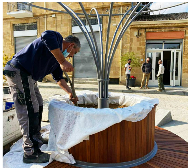
Preparations for planting the climbing plants © Cyprus Energy Agency Photo Archive
