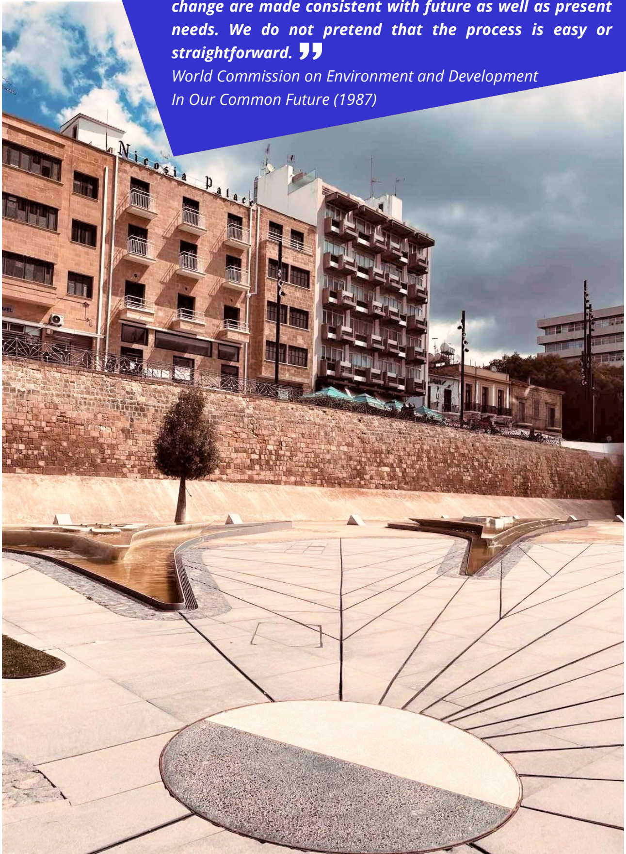
Moat of the Venetian Walls , below Eleftheria Square © Nicosia Municipality Photo Archive
