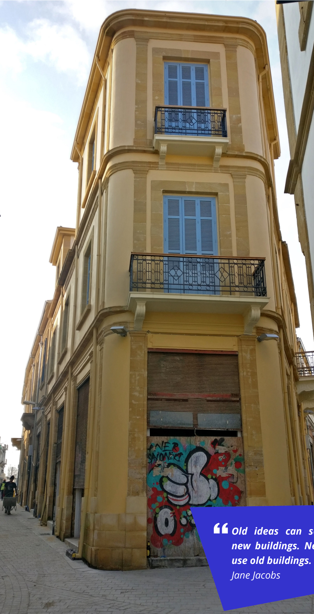
Restoration of buildings in Topali Street. © Cyprus Energy Agency Photo Archive
